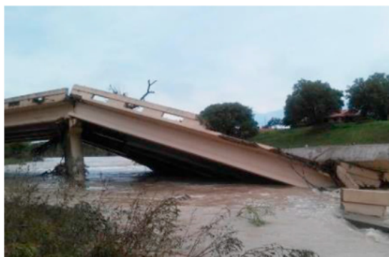
Figure 4. Bridge failures due to hydraulic. (a) Foundation scouring. (b) Bridges submerged by flood. (c) Bridge collapse due to flood
